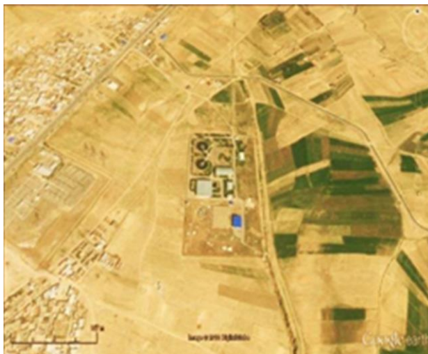
Figure 1. A view of the Ahar Water Treatment Plant
