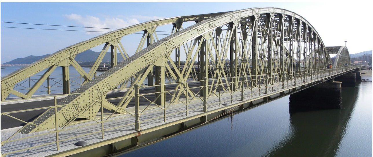
Figure 10. Current status of the refurbished stretches
