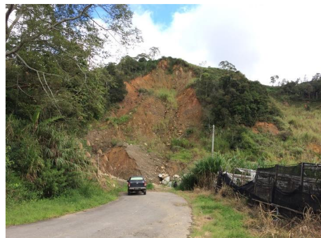
Figure 17. Active rotational landslide on the Mesilau riverbank
