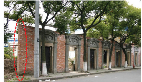
Figure 23. The setting akin to a historic backdrop designed by Deng Kunyan in the Bingjiang Creative Industry Park, photo by the author, 2007
