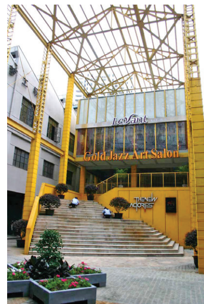
Figure 17. Iron-cast structures in the Er Dongqiang Art Centre in Tianzifang, photo by the author, 2007
