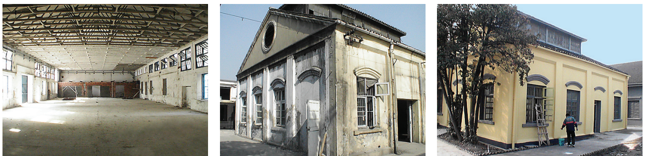
Figure 31. Improper application of new color paints to the preserved historic buildings, photo from www.cg2577.com
