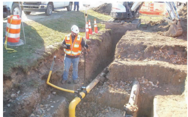
Figure 3. Surveyor recording GNSS observation on a gas main in Michigan, United States.
