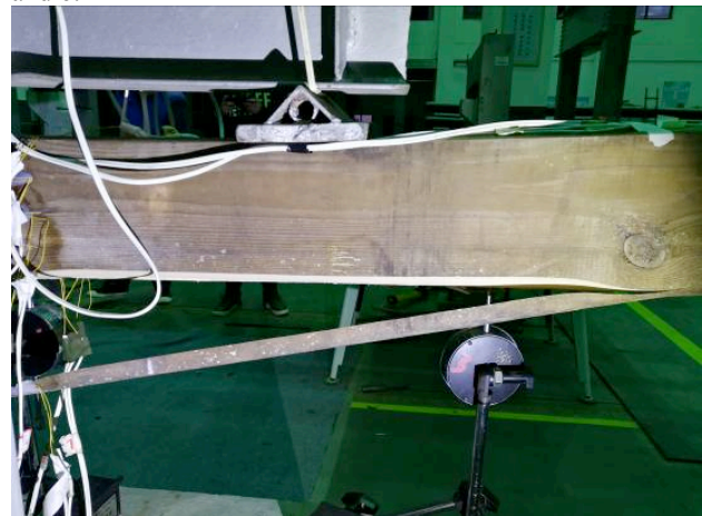
(a) Cracking at beam bottom
