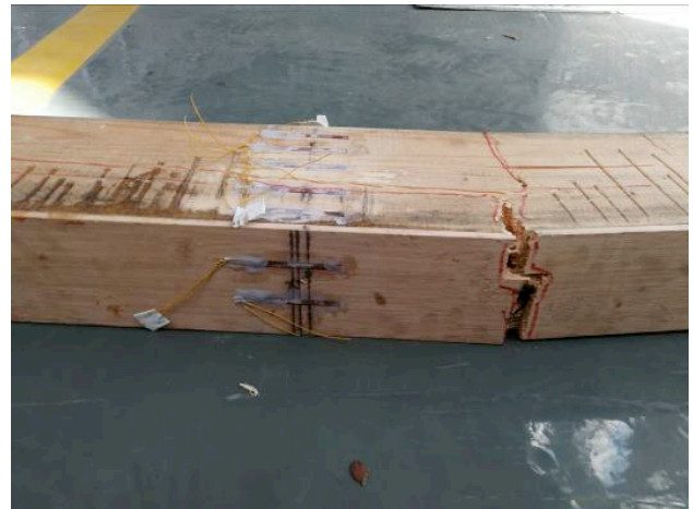
(b) Tensile failure of beam bottom
