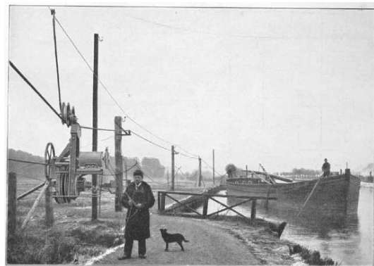
Figure 7. Example of an unmanned electric tractor system designed by Richard Lamb at the end of the 19th century [6].
