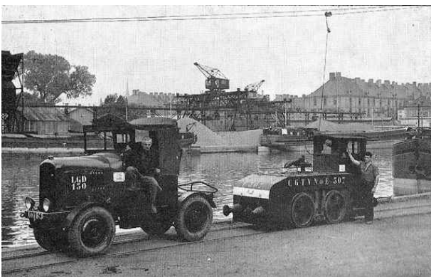
Figure 5. The truck and rail tractor used to move the barges [6].
