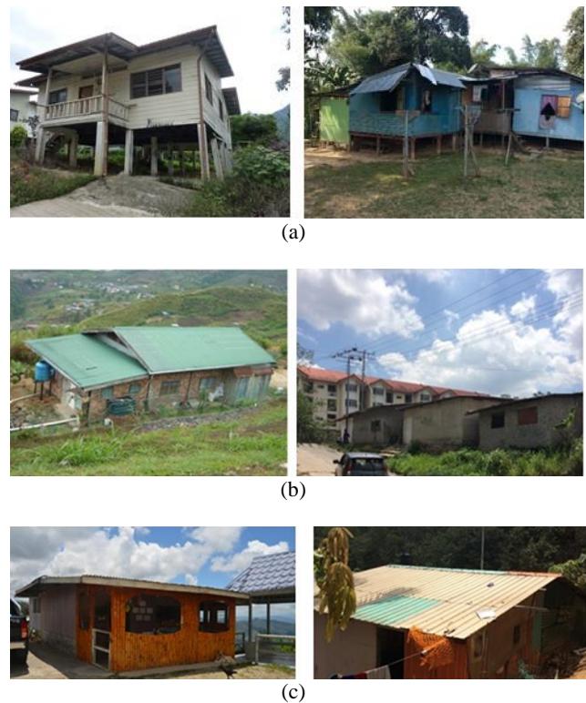
Figure 4. Examples for poor wood/zinc/cement-board building with pillar (a), Poor single storey confined brick masonry building (b) and poor single storey wood/zinc/cement-board building (c) for Kundasang (left) and Kota Kinabalu (right) respectively
