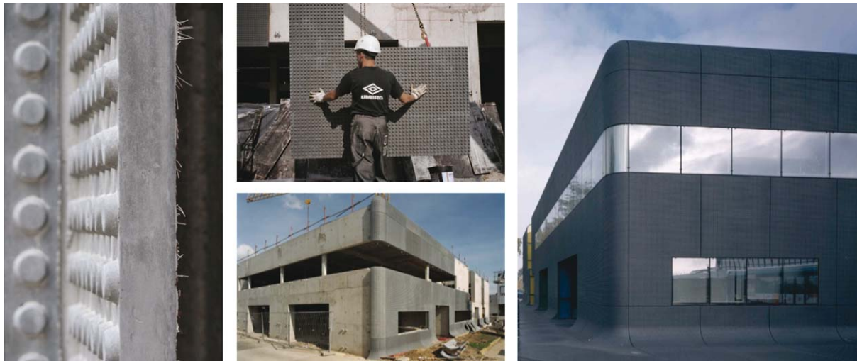
Fig. 1. Examples of the UHPC fibre-reinforced cladding in a curtain wall (Szolyd, 2014).
