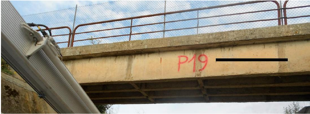
Figure 3: T2 type bridge.
