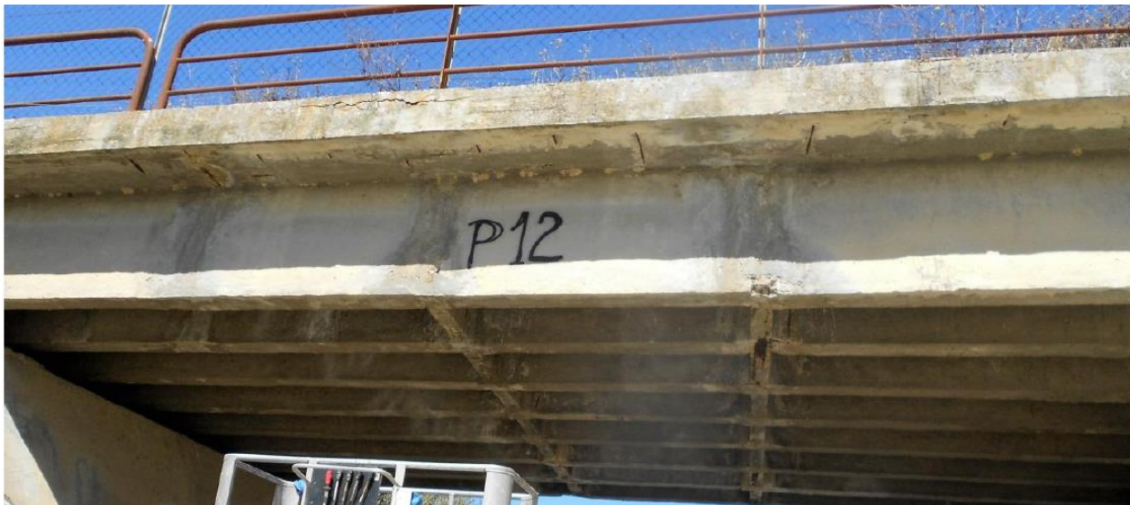
Figure 4: T3 type bridge.
