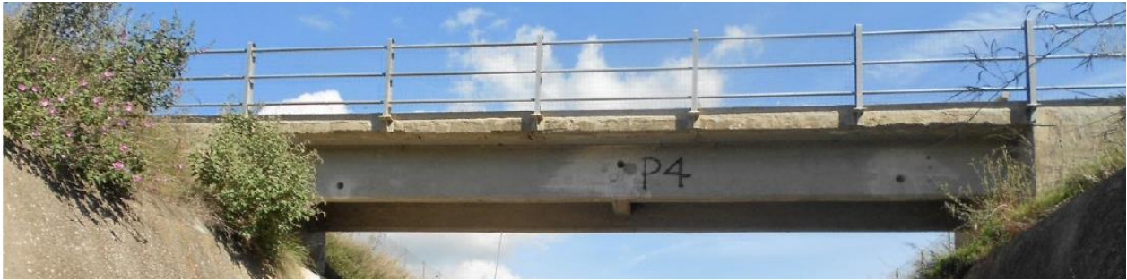
Figure 2: T1 type bridge.
