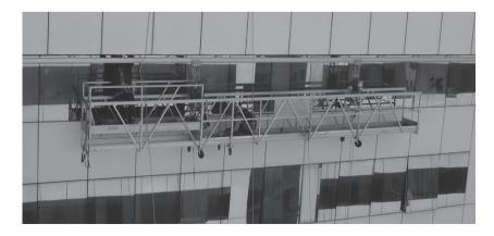
Fig. 2. Building maintenance unit. Source: Rostek.
