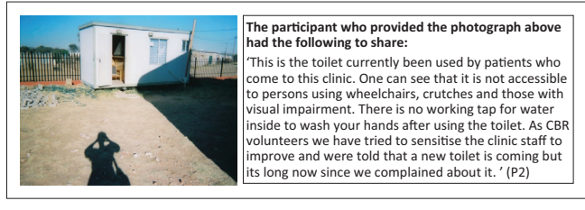
FIGURE 10: Inaccessible public buildings. Need for accessible toilet at local clinic.
