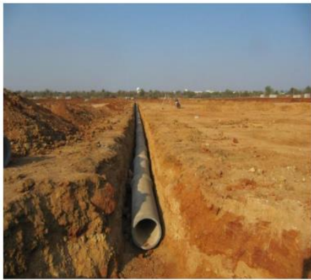
Figure 8. Sample image of sub soil drainage.
