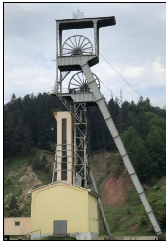
Figure 5. Aninoasa mine extraction tower (2018) Source: Cristina Merciu
