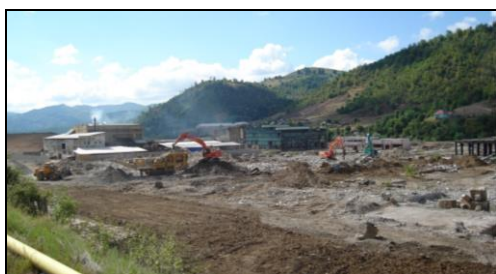
Figure 1. Decommissioning of the former S.C. Ampelum S.A. (2009) Source: Elena Bogan
