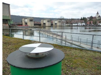
Figure 1. The ship lock (monitoring object) and a photogrammetric control point marked with a forced-centering checkerboard target on a pillar in the foreground.
