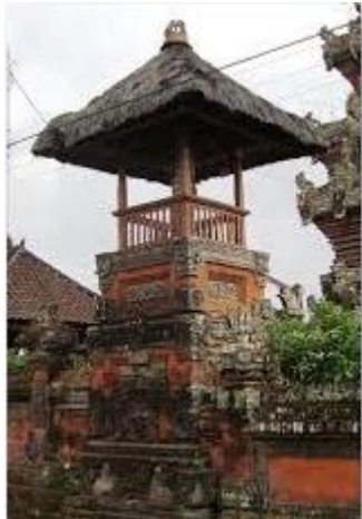
Picture 1. Kulkul building in front of temple building
