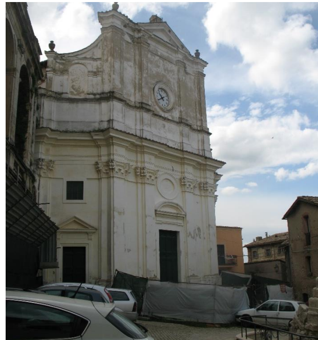
Figure 2. Current photo of the church's facade of Maria SS. Assunta in Cielo, located in Cantalupo in Sabina (RI).
