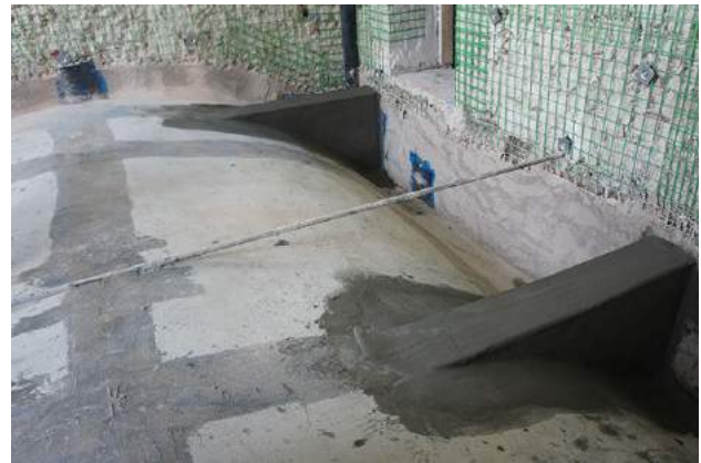
Figure 3: Reinforcement of the vaulting ceilings with carbon fiber bands and solid brick spurs.
