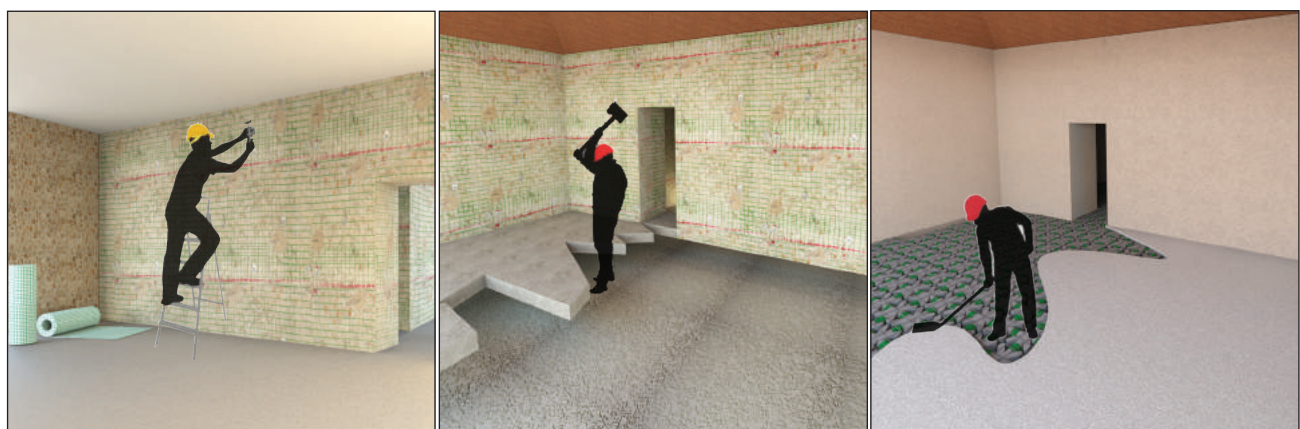
Figure 8: From the left, application of fiberglass- screed removal
