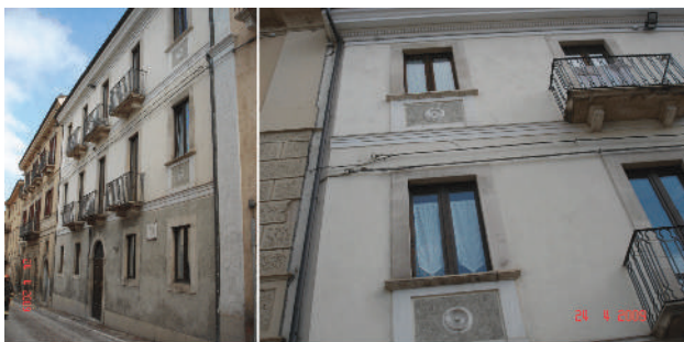
Figure 1: Pre-working condition, after earthquake 2009
