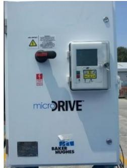
**Gambar 4. Variable Speed Drive (VSD)**
