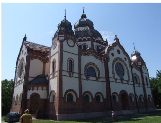
Figure 1 – Synagogue after the restoration of the outer shell in 2016 (photo by: Aladžić Viktorija)
