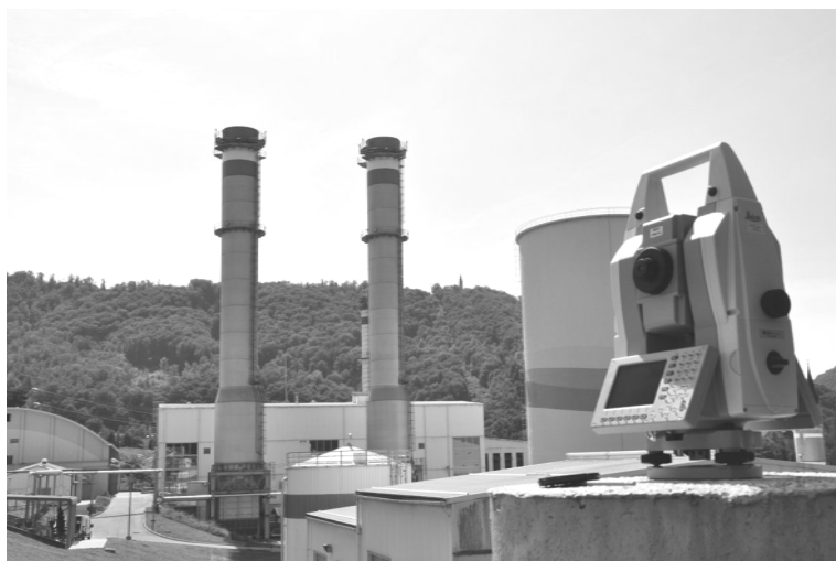
Figure 3. Chimneys of the Thermal power plant Brestanica, Slovenia.
