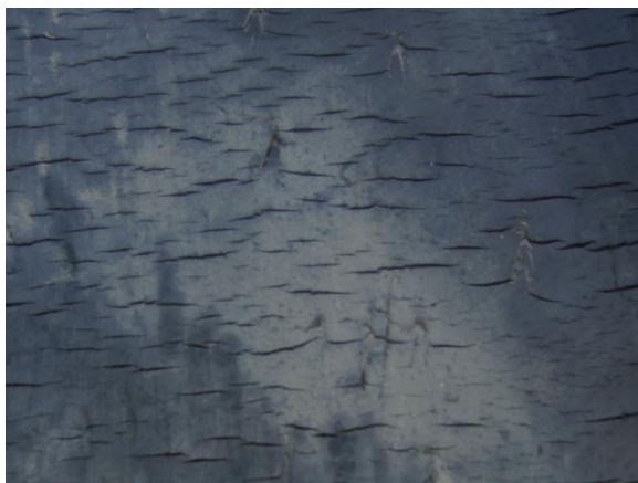
a) network of cracks on the carrier face
