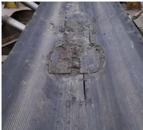
Figure 3. The longitudinal splicing of the conveyor belt
