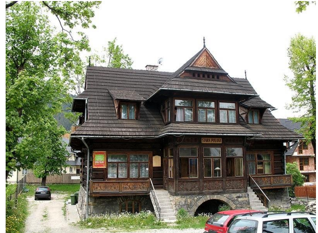
Fig. 2. A photo of the Stara Polana building in Zakopane (own source)
