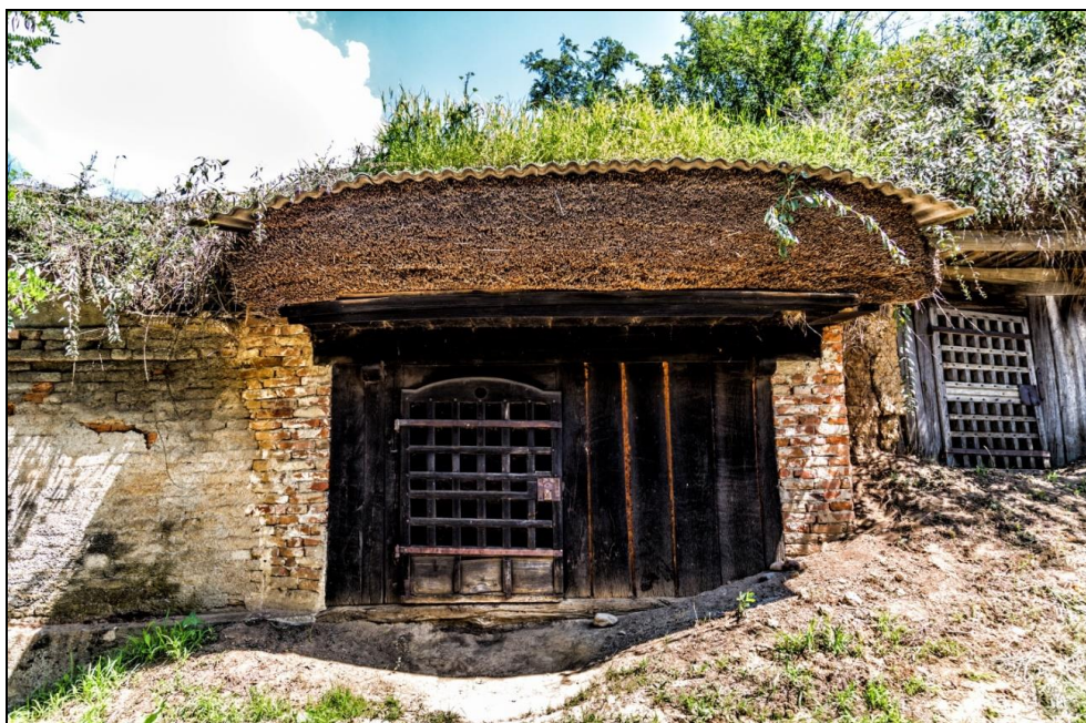
Figure 6. Brick cellar Salacea
