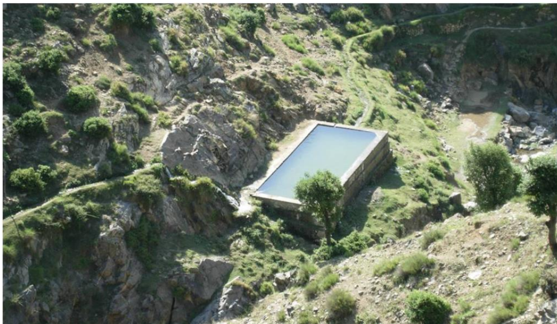
Figure 5. Reservoir for the storage of surplus water discharge from springs
