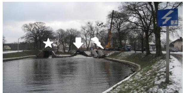
Fig. 2. Construction of the Small hydroelectric power plant Łochowo.
