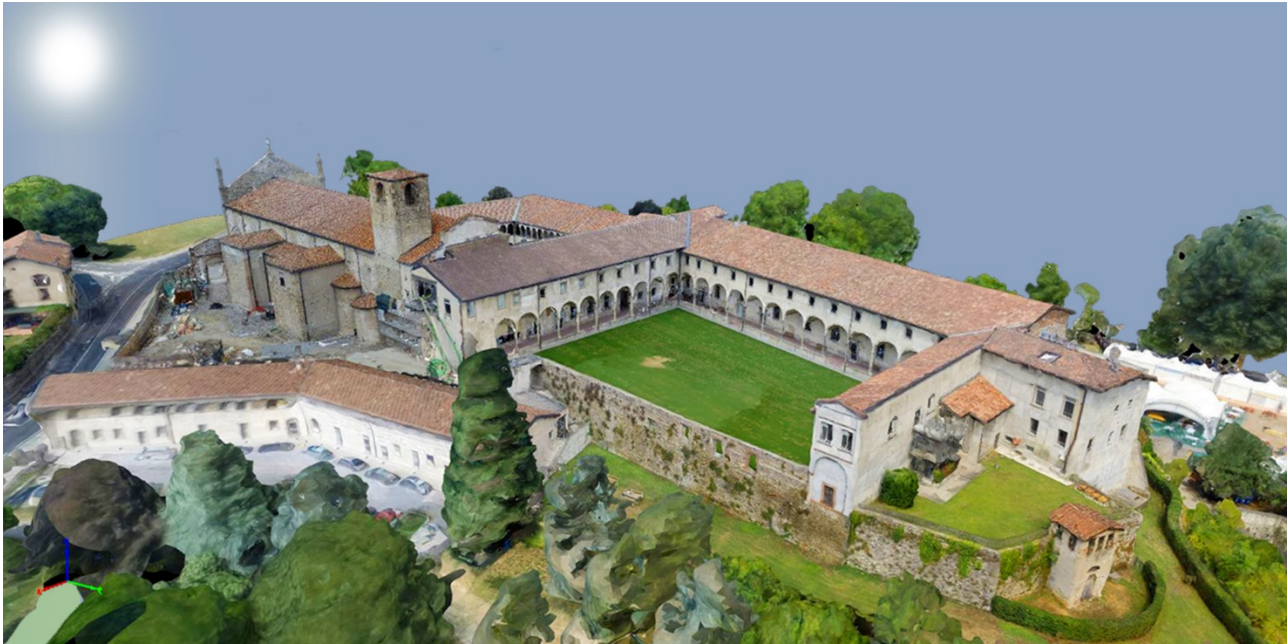
Figure 8. The complex of Sant'Agostino acquired from drone (summer 2015): a bird's eye view of the 3D model.
