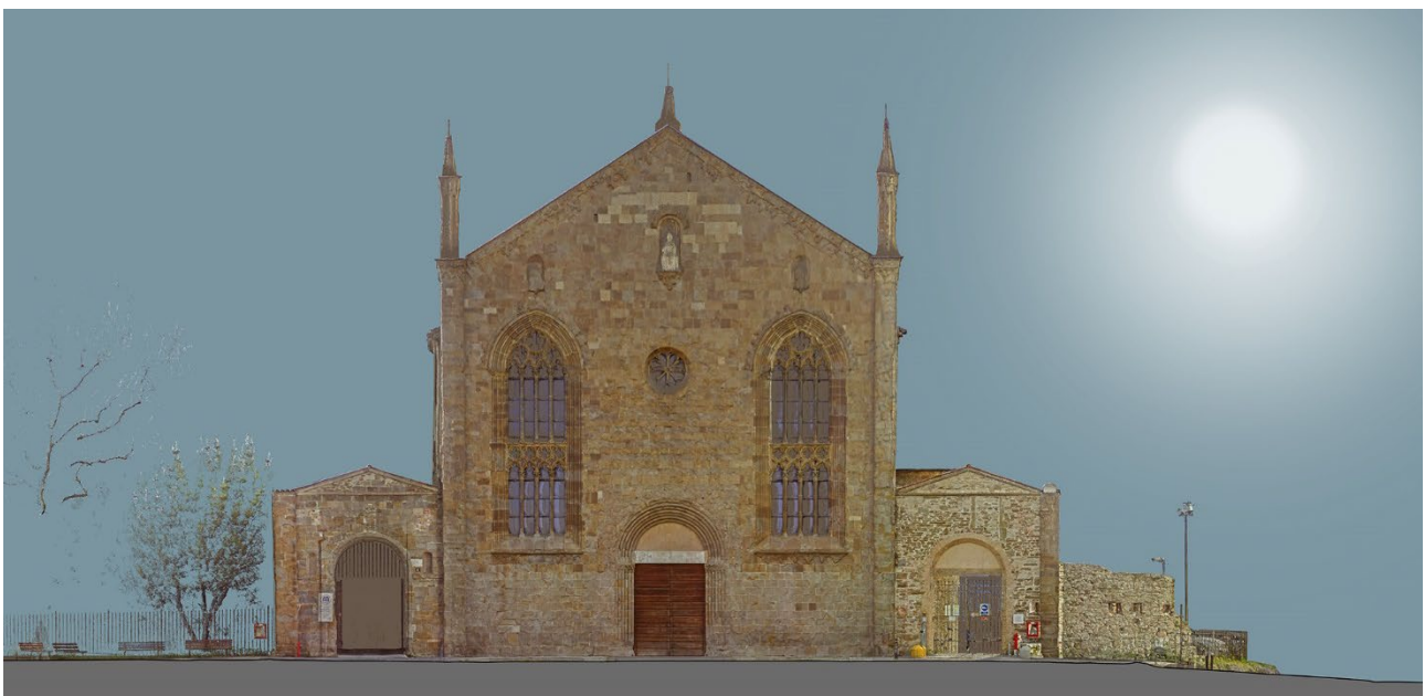
Figure 4. The façade of the church of Sant'Agostino after the restoration: the orthographic projection of the points cloud.
