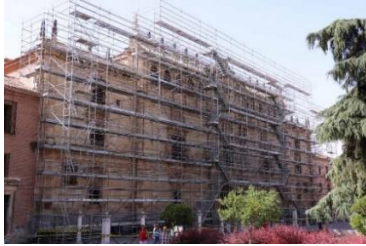
Figure 1: Façade University of Alcala. Restoration, 2017.
