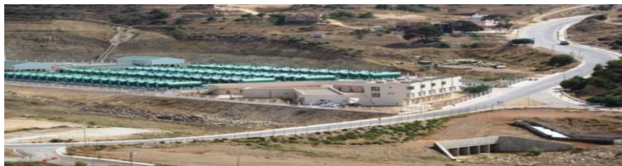
Fig. 1. Desalination Station-Honaïne – Tlemcen [28].
