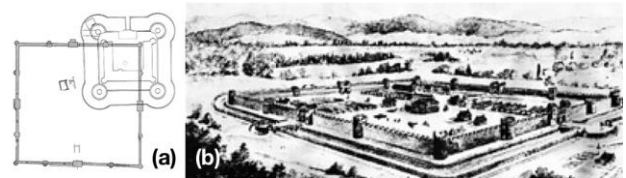
Figure 6. Graphical data of the castellum; (a) Theoretical plan of the castellum and the castle of Horbourg-Wihr, prepared by E.A. Herrensneider (1894); (b) Horbourg-Wihr's castellum elevation, according to architect C. Winkler (1905).
