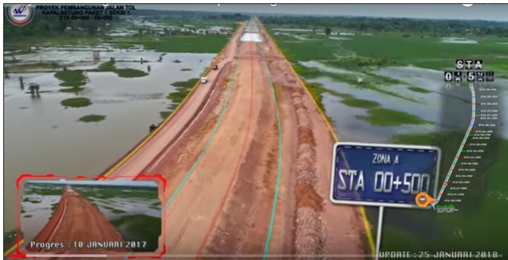
Figure 1 – Construction of the Kapal Betung toll road and flooded rice fields
