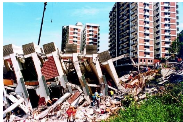
Figure 2: Image of the collapsed Highland Towers residential building in Ampang Jaya in 1993
