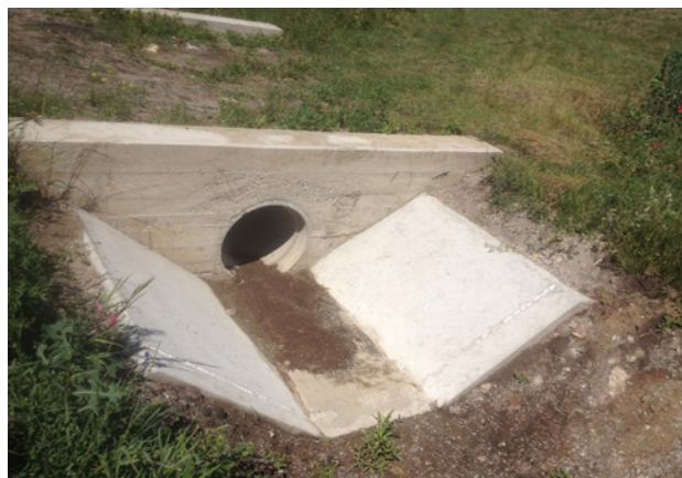
b) Prefabricated tubular bridges
