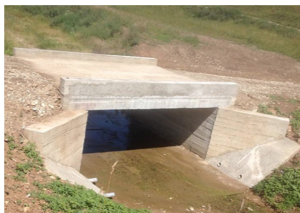
d) Road bridge of concrete
