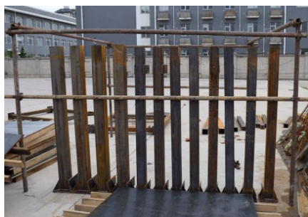
(a) Fabrication of the steel tube
