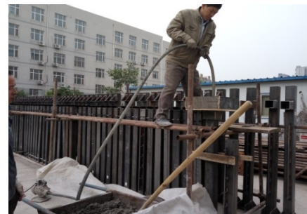
(b) Pouring RAC in the steel tubes
