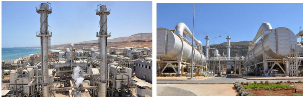
Figure (3). General view of Zuara and Sussa desalination plants each 40,000 m 3 /day.
