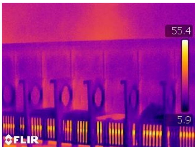
Fig. 15. Convection current caused by static heaters in St. Sava Church.
