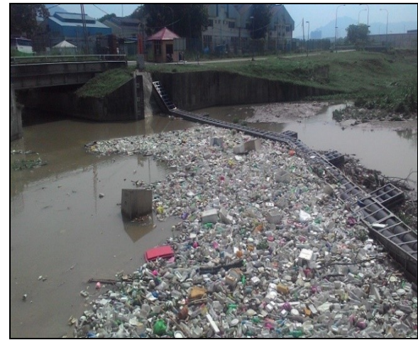
Fig. 2. The accumulation of floatable litter at log boom Sungai Batu
