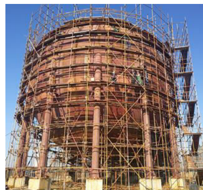
Fig. 1. Spherical tank in the construction.
