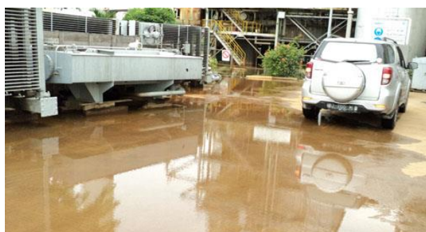
Fig. 19. Documentation of flooding from tidal inundation and rain affected building condition due to land subsidence
