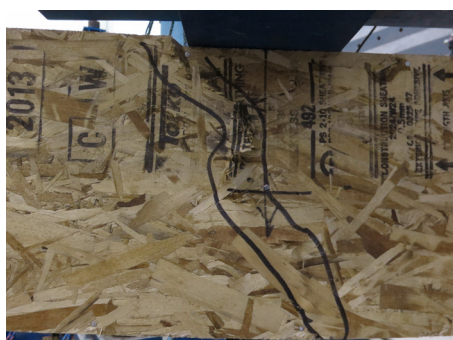
(a) web shear failure
