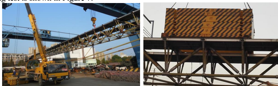
Fig. 7 Loading test photo under intermediate load condition
