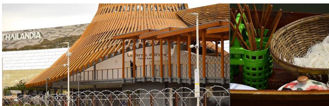
Fig. 5. Thailand pavilion (expo2015.org).
