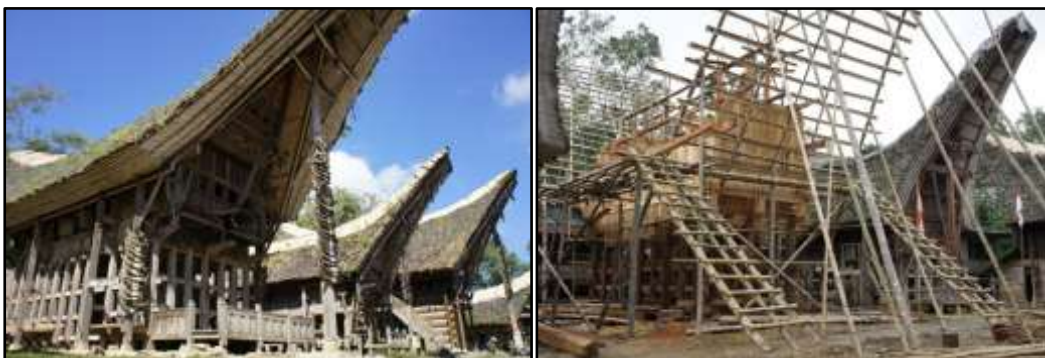
Figure 1. Torajan Tongkonan. Figure 2. Torajan Tongkonan in construction. (copyright authors)
