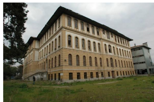
Image 1. General view of the south façade [6]
