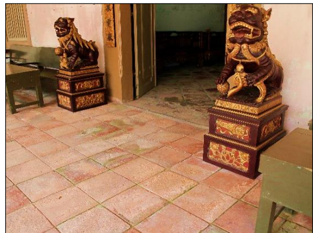
Figure 12. The original Terracotta Brick floor to the Altar Room (Source: Putranto & Pradnyawan, 2017)
