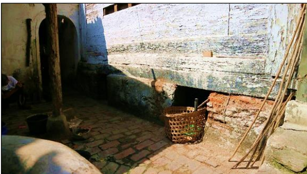
Figure 17. Hollow under the house is one of the characteristics of Chinese house (Source: Putranto & Pradnyawan, 2017 )
