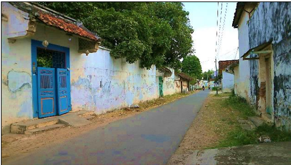
Figure 15. Walls around a Chinese House in Karangturi Region. (Source: Putranto & Pradnyawan, 2017 )
