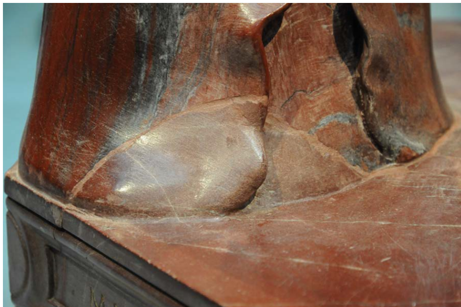
Figure 44. S-1: Join between the antique part at the base connecting the front of the support to the plinth.
