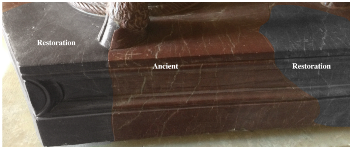
Figure 51. P-8: The left-side panel features an ancient fragment that also continues onto the ground of the plinth above. It appears to attach to the goat's left foreleg.
