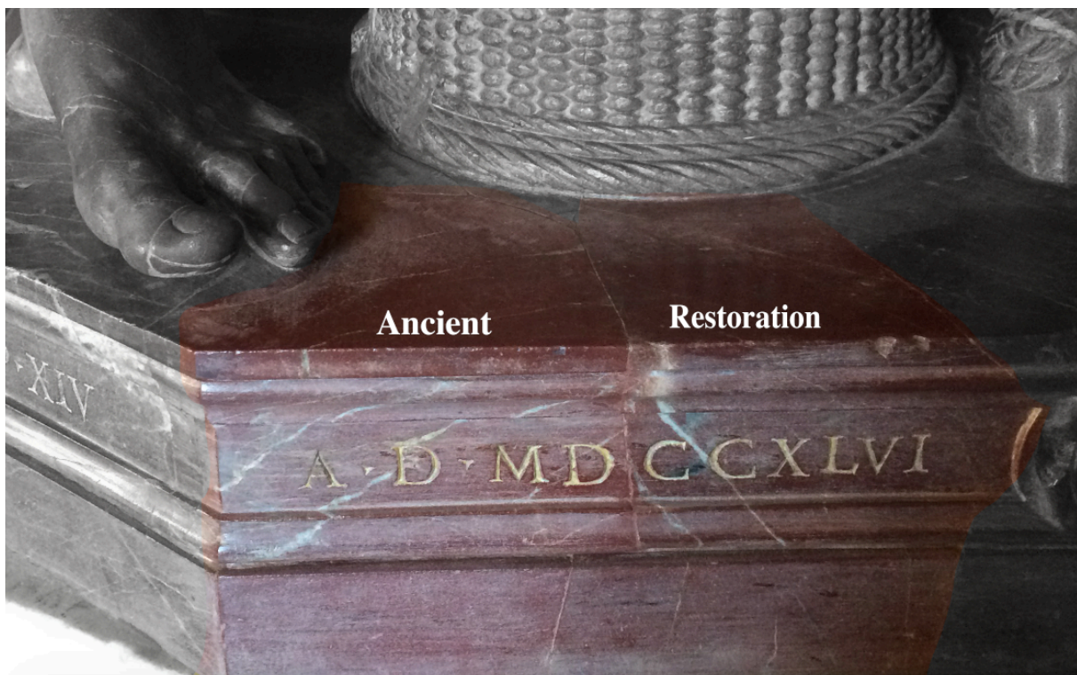
Figure 45. P-1: The front left (proper) panel, which reads "A D MDCCXLVI" features a seam between "MD" and "CC" that delineates the ancient (P-1) and modern (note the grey veins running through the marble of restoration).
