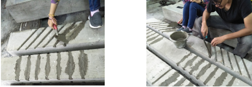
Fig. 2. The installation process of NSM steel bars.
