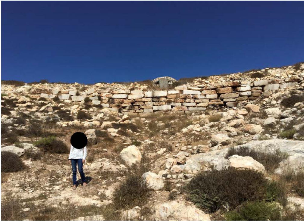
Figure 3: The southern wall bordering the terraces of a new agricultural pioneer front between Yasid and Beit Imrin. It corresponds to exploitation 2 represented in Figure 2. Source: authors.
