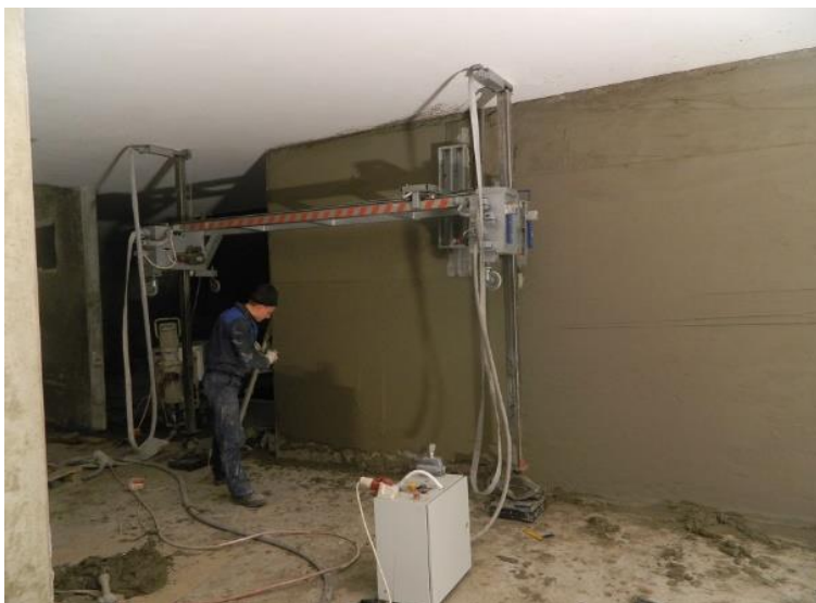
Fig. 1. Plasterer robot PlasteRUS Foreman.
