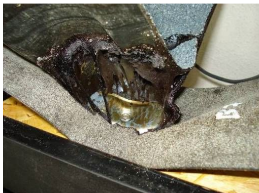
Fig. 3. Typical damage of joint of specimen B. Source: [1].
