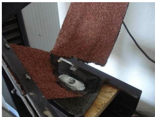
Fig. 4. Opened joint of specimen C without deformation of anchoring element. Source: [1].
